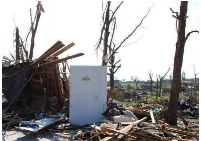
This In-residence Safe Room, (manufactured by a NSSA member) located in a garage protected two people (Joplin, MO).
